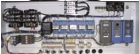
Photographed before final insulation.
